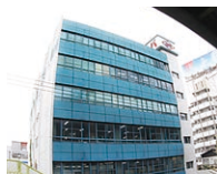
本社／本社営業部 Head Office / Head Office Sales Department
